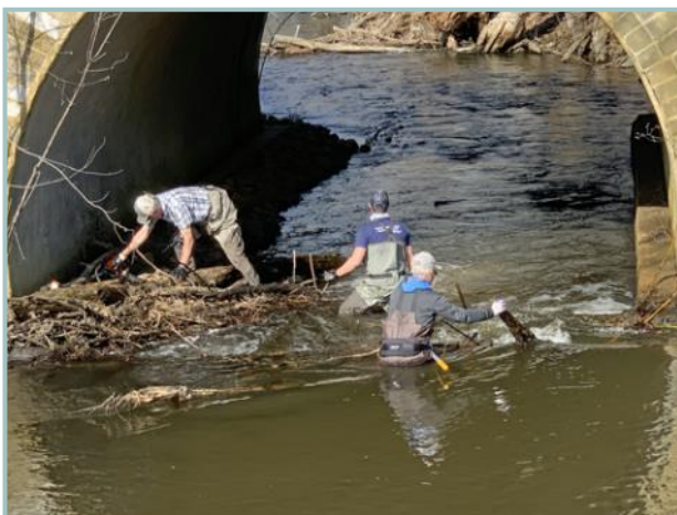
Before and after at the bridge. Clearing out the blockage led to the water level dropping two feet. Well done, crews!
